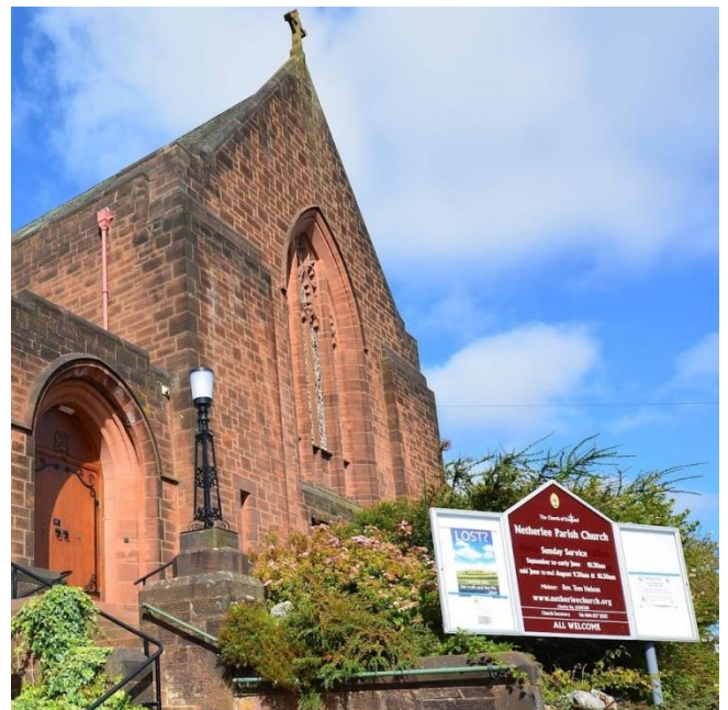
Main Door on Ormonde Avenue
