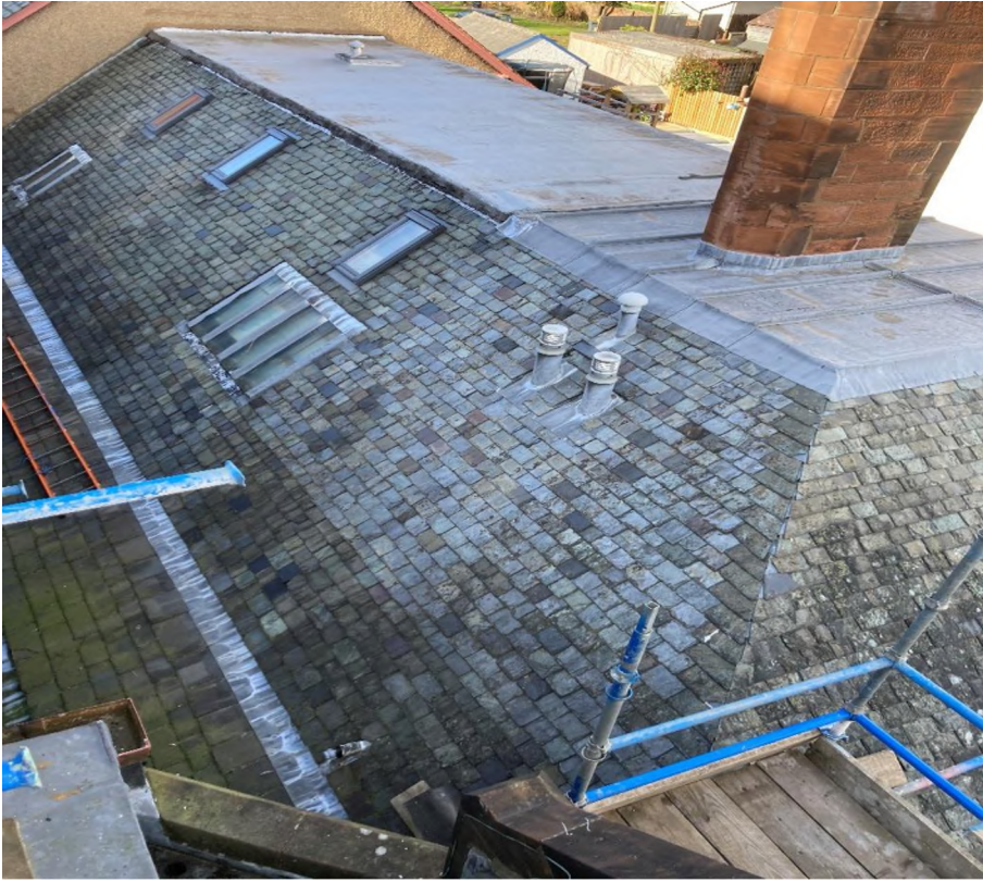
Roof view showing lead & bitumen, slates and 2 elderly skylights
