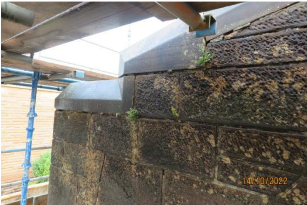
Above stripping underway Below gaps in stonework and growing vegetation
